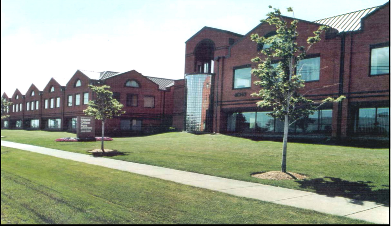
View From Maple Road
