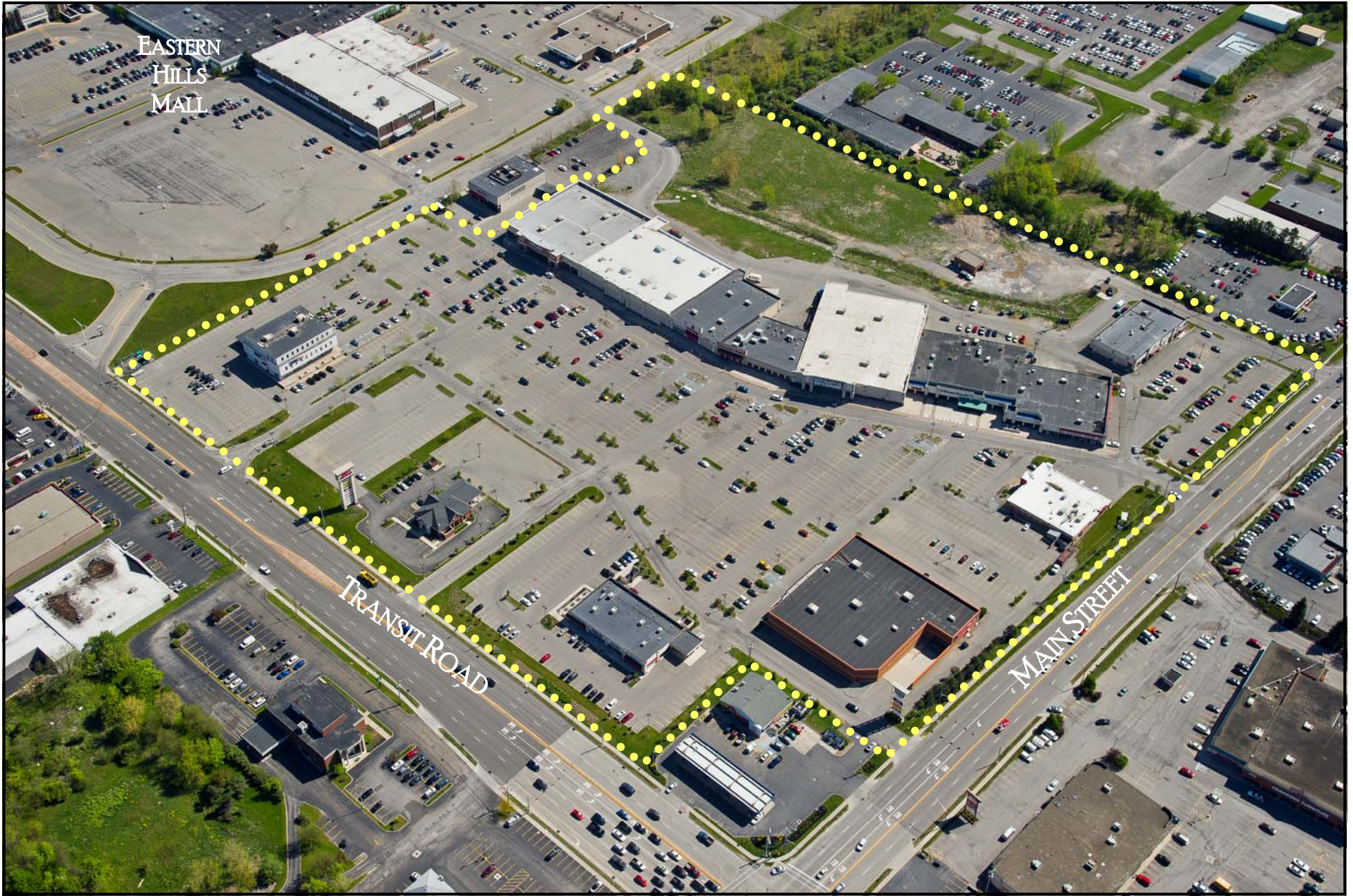
SHOPS AT MAIN/TRANSIT ~ CLARENCE, NEW YORK
